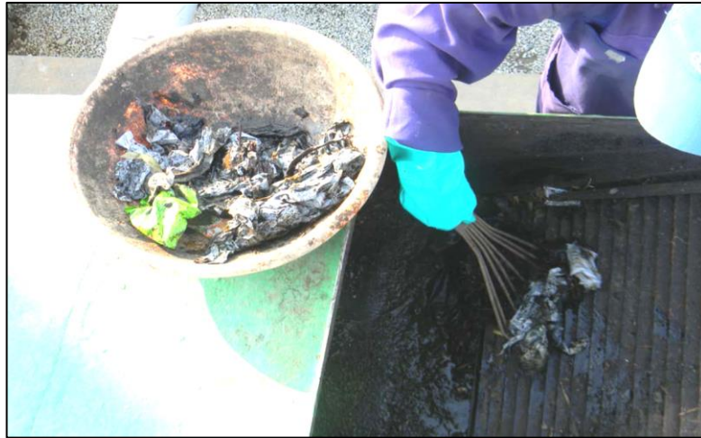
Figure 5: Showing cleaning of screens
